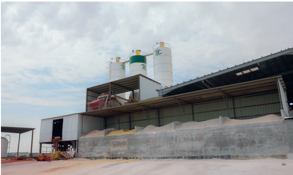
Production site of Riyadh Kingdom Concrete Products Al Ahsa
