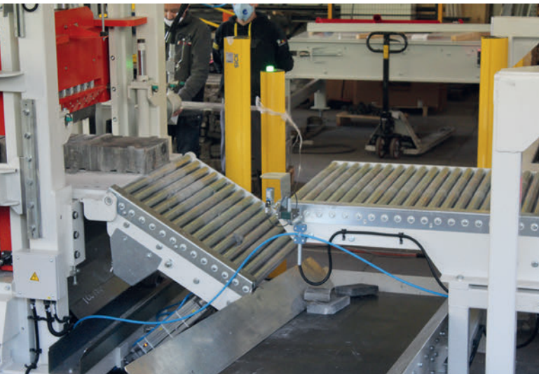
Quality control area
