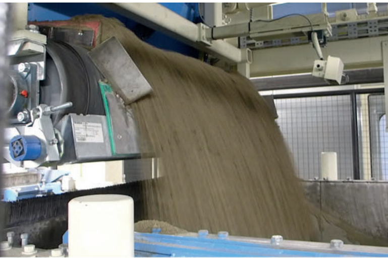
Filling box feeding via dosing belt.
