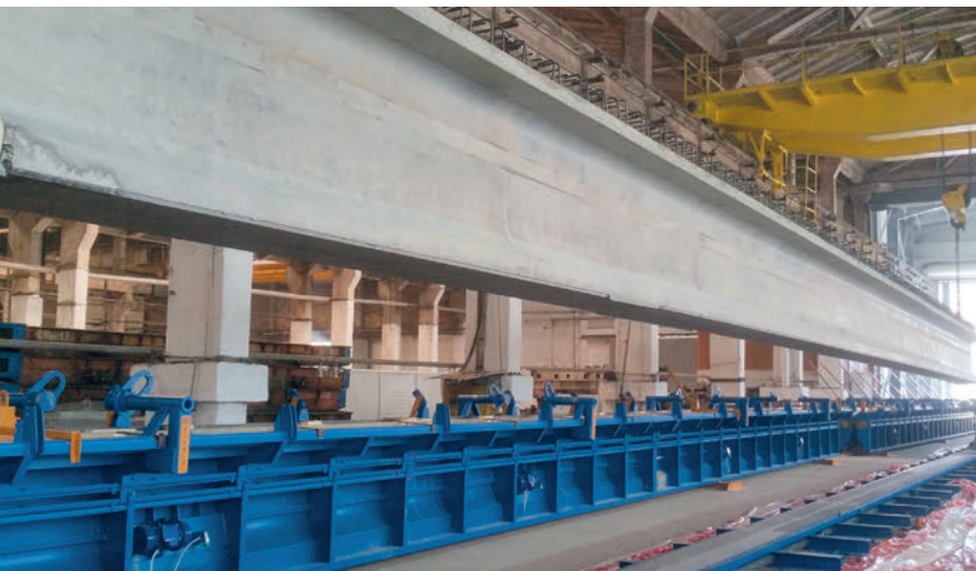
First element lifted from mould
