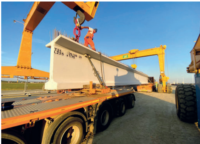
Transport of a bridge girder
