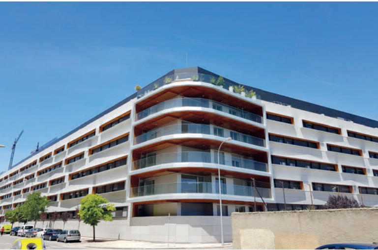
Isla de Arosa: 7,500 m 2 white non-structural skin, thickness: 10-20 mm
