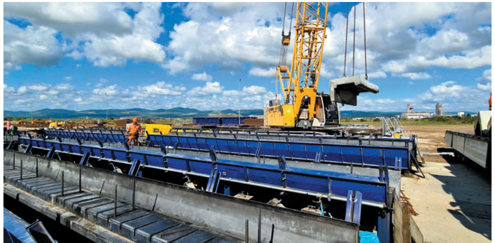
Mould for the production of parapets
