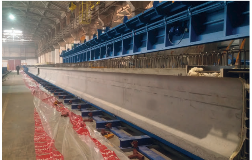
Side mould lifted and demoulded first concrete element
