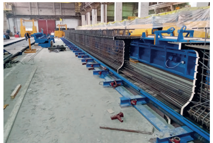
Preparation for the first pouring process
