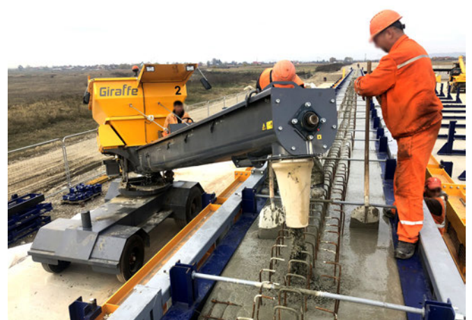
Pouring of the concrete into the mould using Giraffe vehicle
