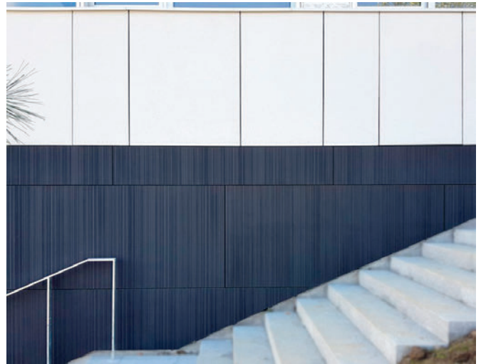
German College of Bilbao: 1,100 m 2 textured skin and 1,100 m 2 pure white panelling, thickness: 14-16mm
