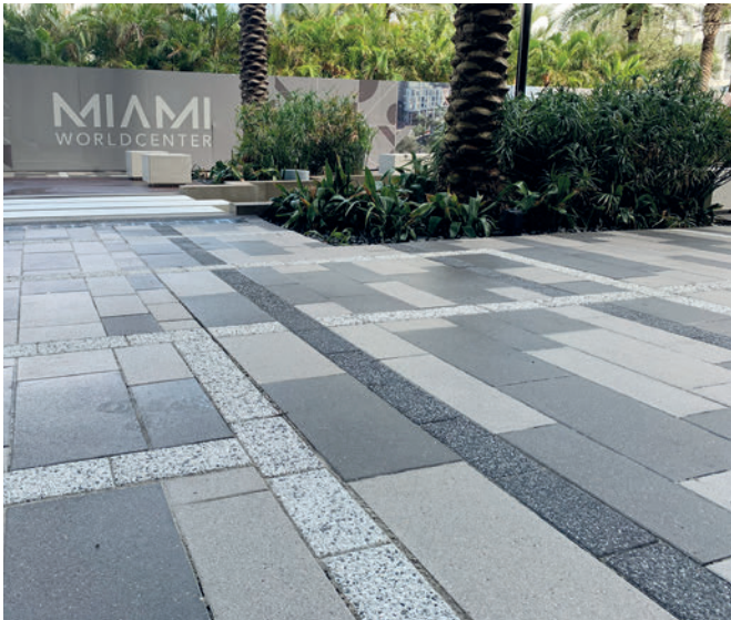
Laying Wausau pavers
