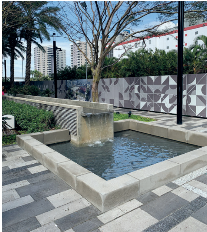
Laying Wausau pavers
