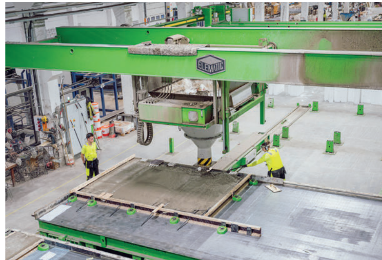
Casting concrete elements
