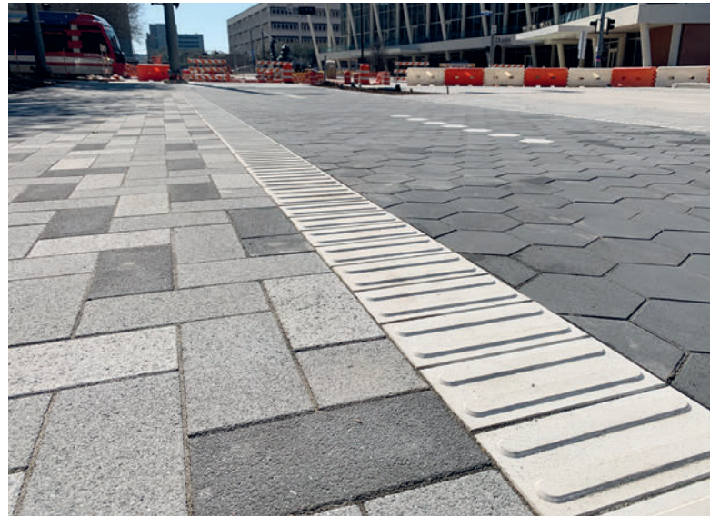
Bagby Street: Stone installation pedestrian and bicycle area
