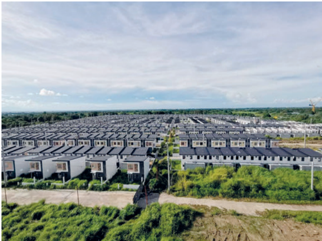
Megawide is planning to add two projects every year, as they see an increasing need in the future.
