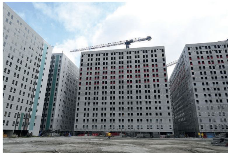
14-storey mid-rise affordable housing built with 90% precast
