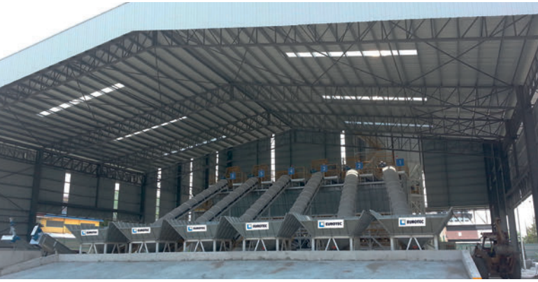
The enclosed warehouse reduces noise and dust emissions
