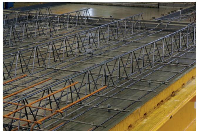
Ready for concreting
