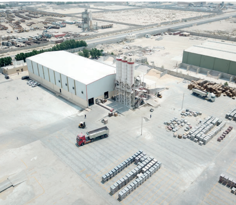
Bird's-eye view of the new production hall
