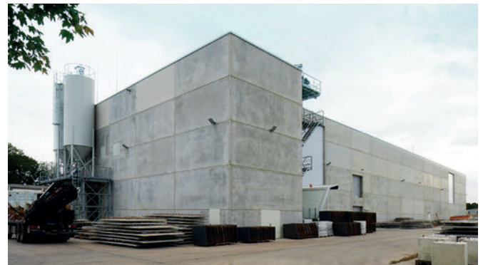
The new production hall and mixing plant
