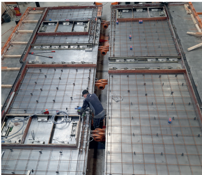
Butterfly Formwork in unfolded position - Horizontal preparation
