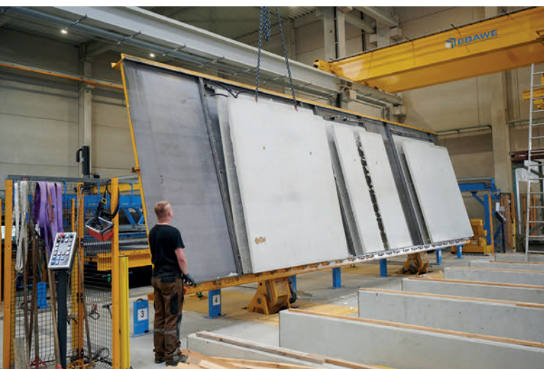
Vertical lifting of the double walls at the tilting station
