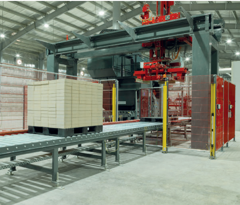
The stone packages being finished are transported by the heavy-duty conveyor to the LPU layer stacker.
