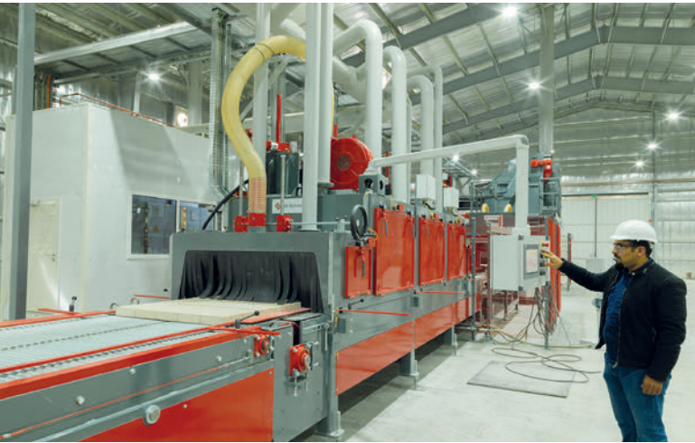
The curling machine has its own control system with operating panel and display.
