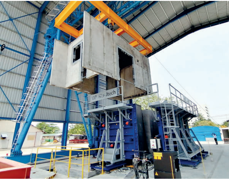
Demoulding of finished elements
