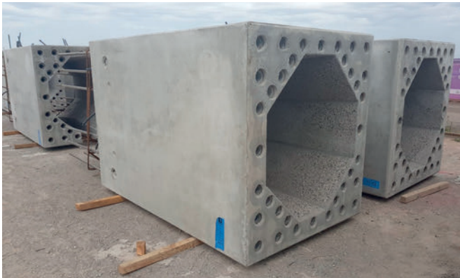
Composite “shell” mega columns used to assist lateral stability of Premier Tower, Melbourne.
