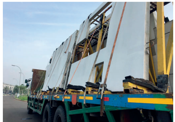
The earthquake tested and safe elements with the cut outs for doors and windows already implemented are transported to the sites.
