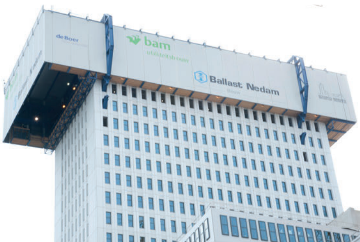
Erasmus Medical Centre, Rotterdam, The Netherlands
