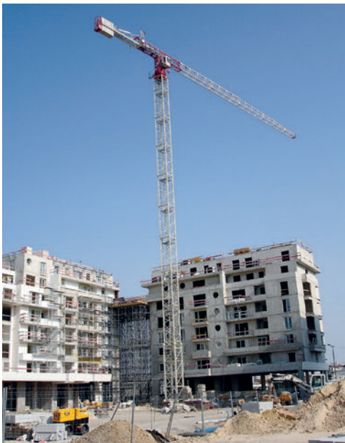
Large panel / wall frame system as a proven precast technology for mass housing projects
