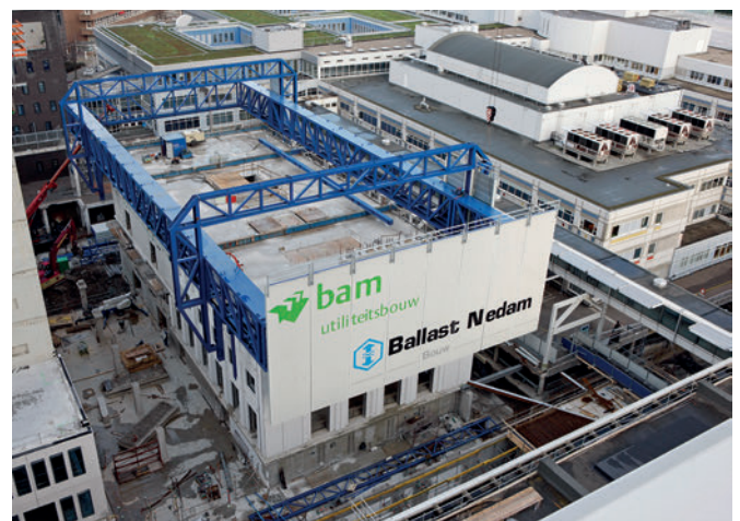
Climbing Shed being assembled
