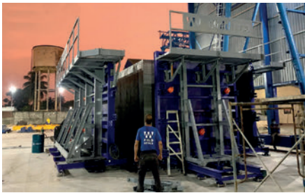
General view of the mould with vibrators
