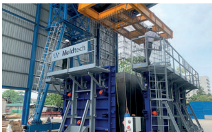
Insertion of reinforcement with lifting beams
