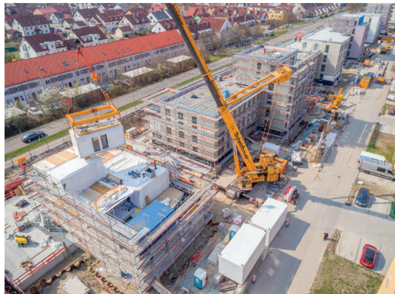
Construction of a modular building
