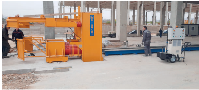
Strands anchoring structure
