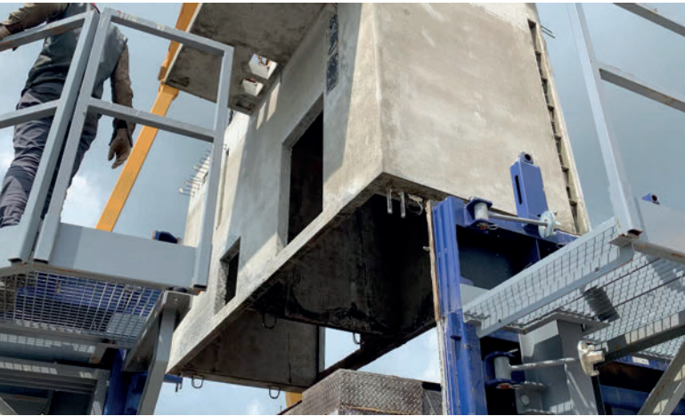
Demoulding of a casted element
