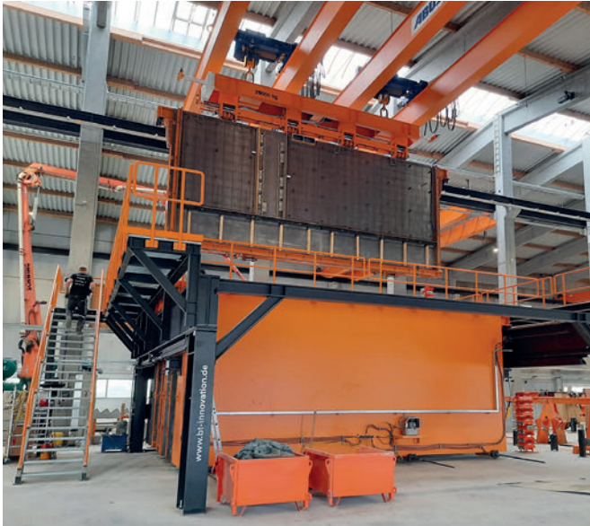
Mounting the Butterfly Formwork® in the battery mould
