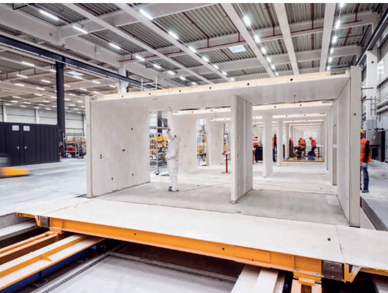
Production of room cells for modular construction
