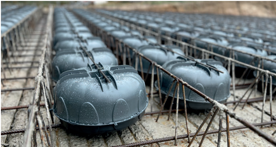
Fig. 4: Semi-precaster slab with void formers placed on top
