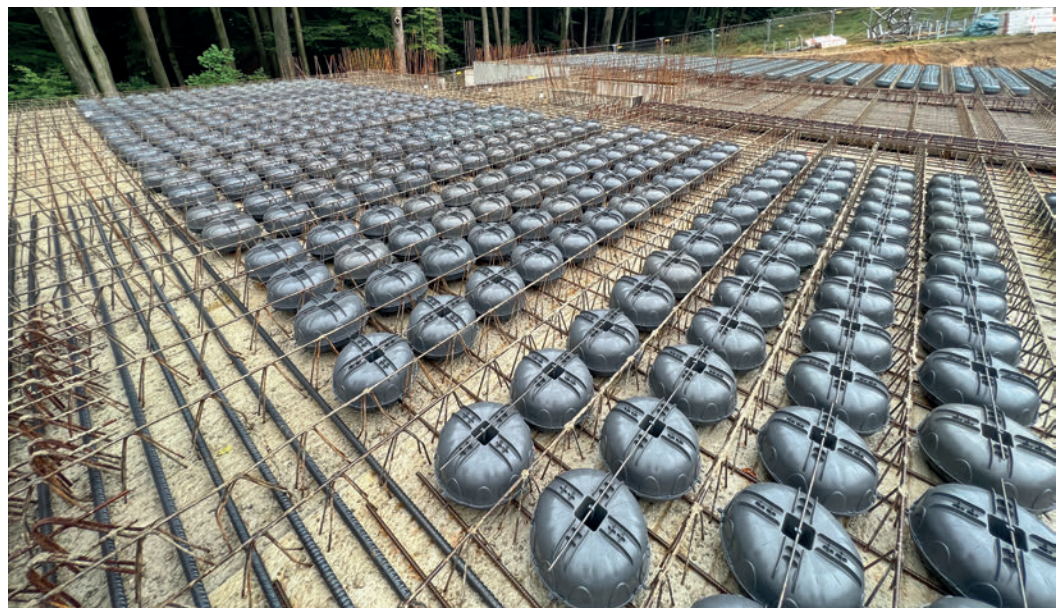
Fig. 7: Installed semi-precast elements with transverse reinforcement and Unidome void formers
