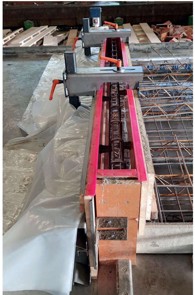
MST extension for the production of upstands
