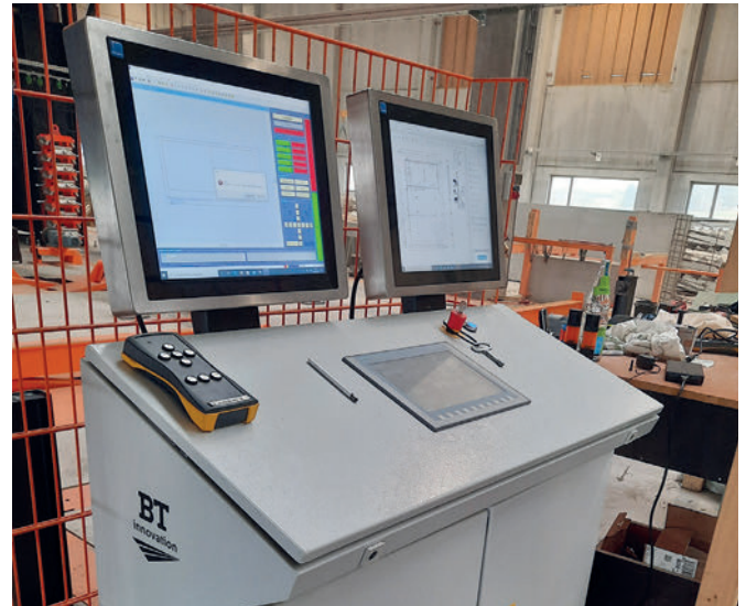
Control point for unfolding and folding station and laser projectors
