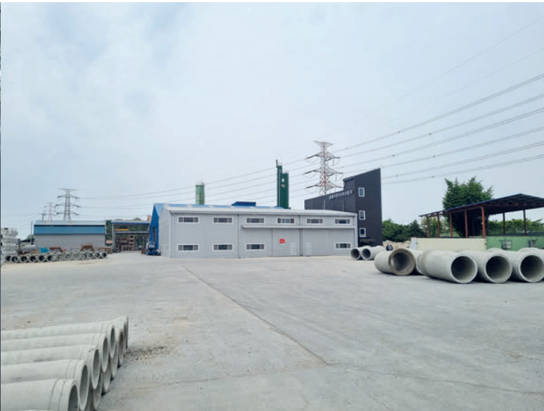
The Hong-Ik Co. Ltd. facility in Seoul, South Korea
