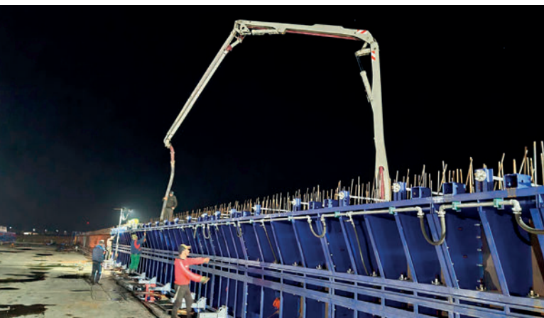
Mould for girders
