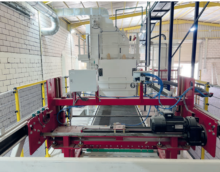
Shotblaster with layer pusher
