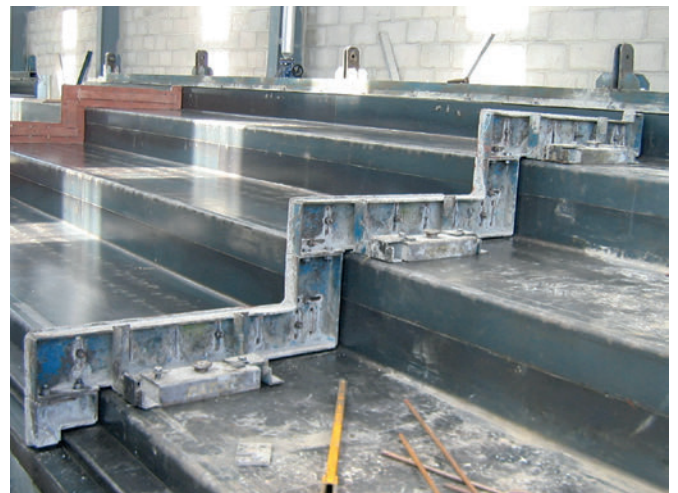
Fastening of stair formwork by means of SPB
