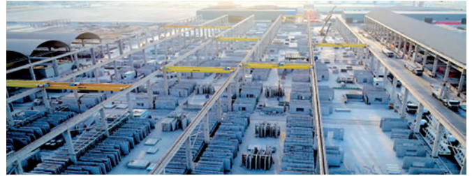
View of Abu Dhabi Precast yard
