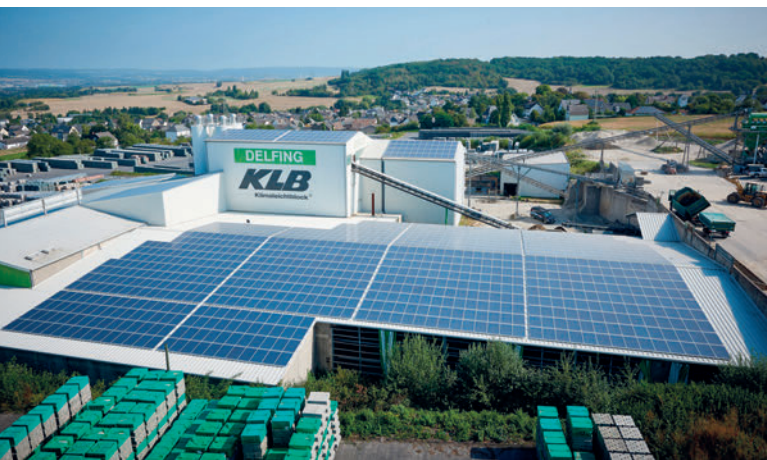
View of part of the large company premises. The roof surfaces are covered with solar modules for sustainable energy generation
