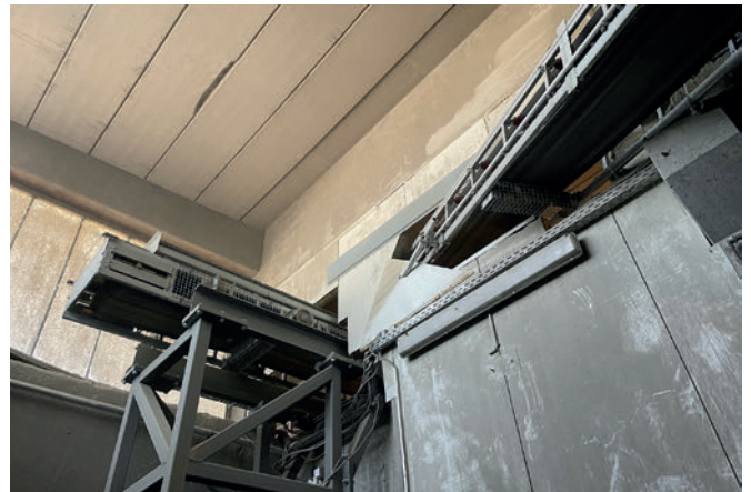
New conveyor belts for concrete transport
