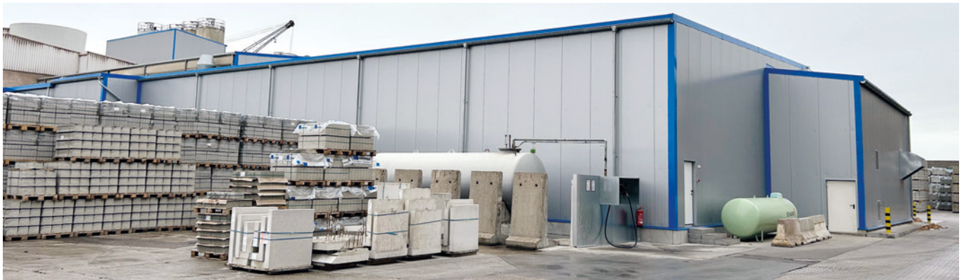
The new large-capacity curing chamber at Kronimus in Heilbronn, Germany.
