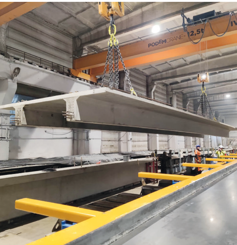
Double T being lifted
