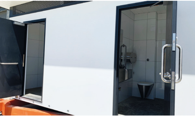
Finished bathroom unit
