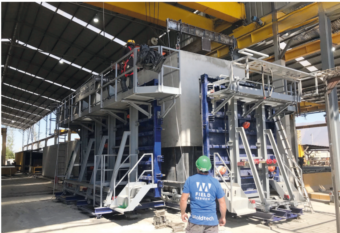
3D modular mold for housing
