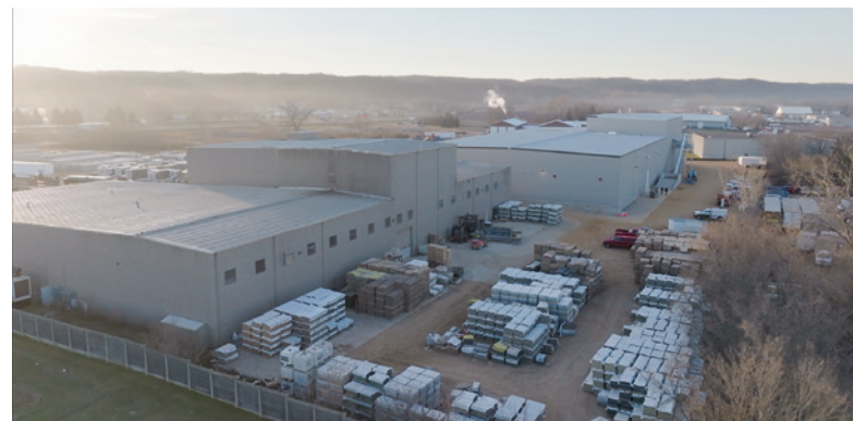
Rochester Concrete Products' new manufacturing plant at their Interlock Concrete location in Jordan MN
