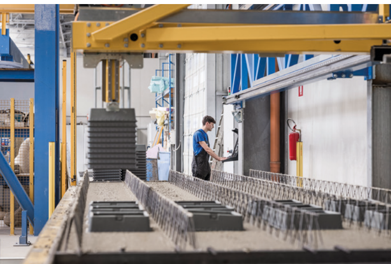
The Box Master places the lower half of the GC box (the GC base) fully automatically in the Green Code Eco Slab® at the plant - this is then completed on building site with the GC top, i.e. the other half.
