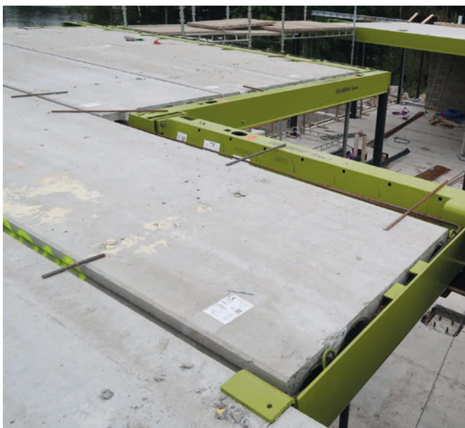
Fig. 5: Hollow-Core slabs installed. Opening in the slab for HVAC (Heating, Ventilation, Air Conditioning) pipes. Petra Slab Hanger supports hollow-core slab.
