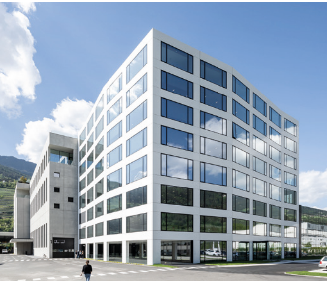
Just a few metres from the Progress Group's new headquarters, their own precast plant is producing precast elements.
