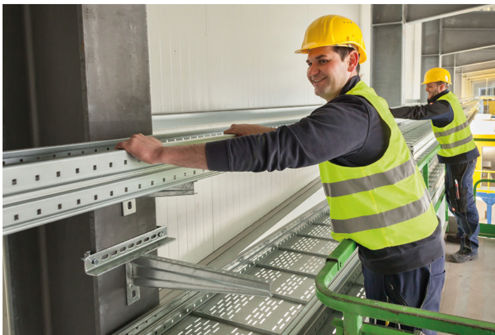
Professional and just-in-time: laying the new cables
