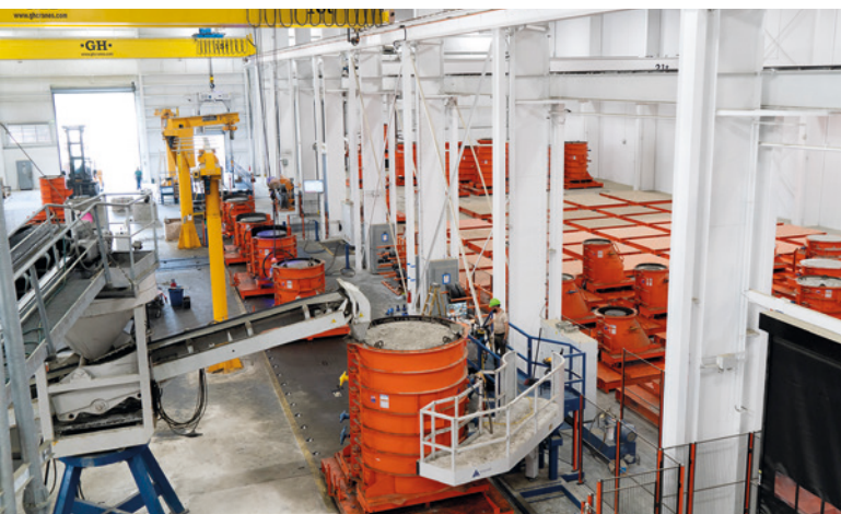
Specialized workstations on the Prima at Tindall Infrastructure in Spartanburg, SC.
