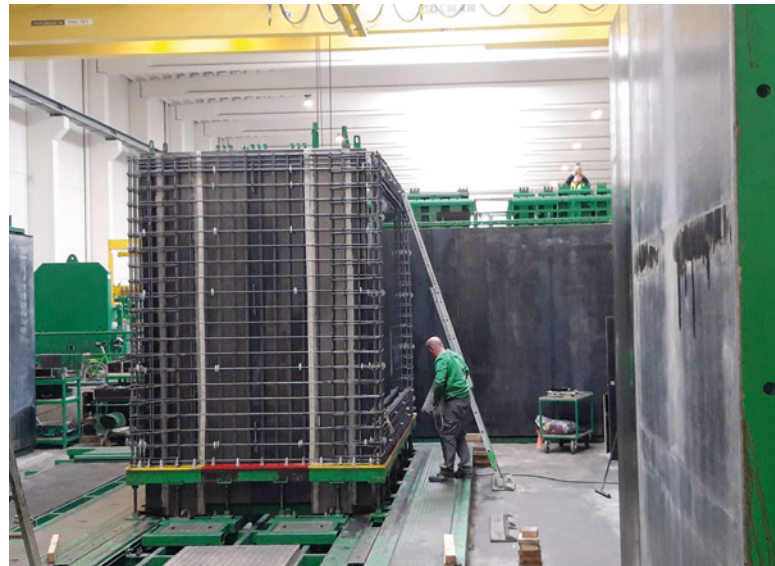
Fixing rebar onto the inner core of the mould
