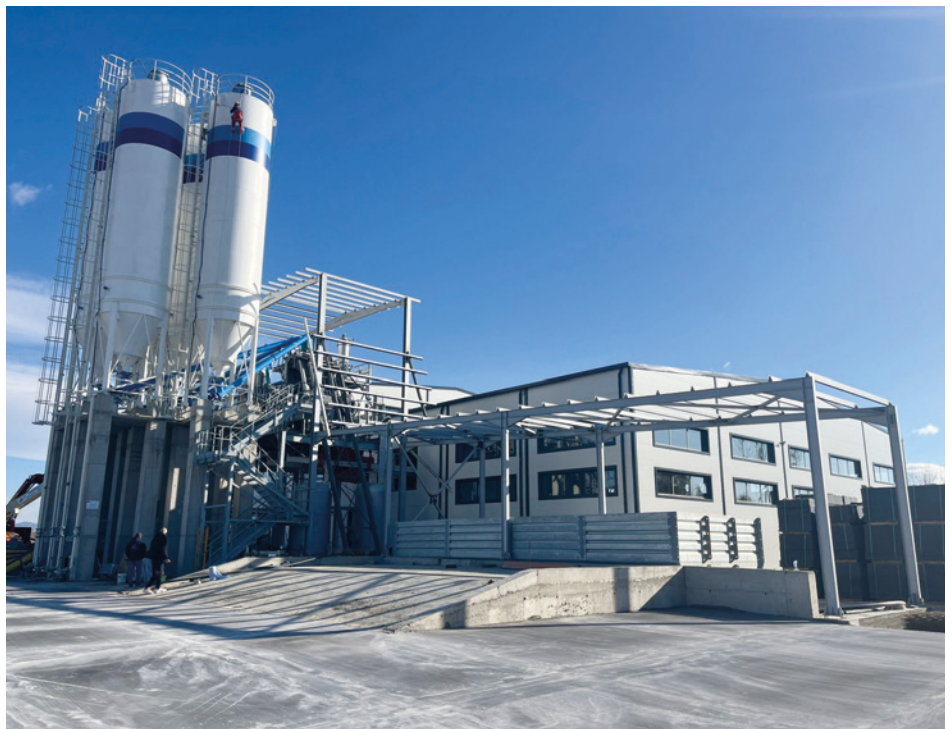
View of the new concrete block production facility in Zhitnitsa
