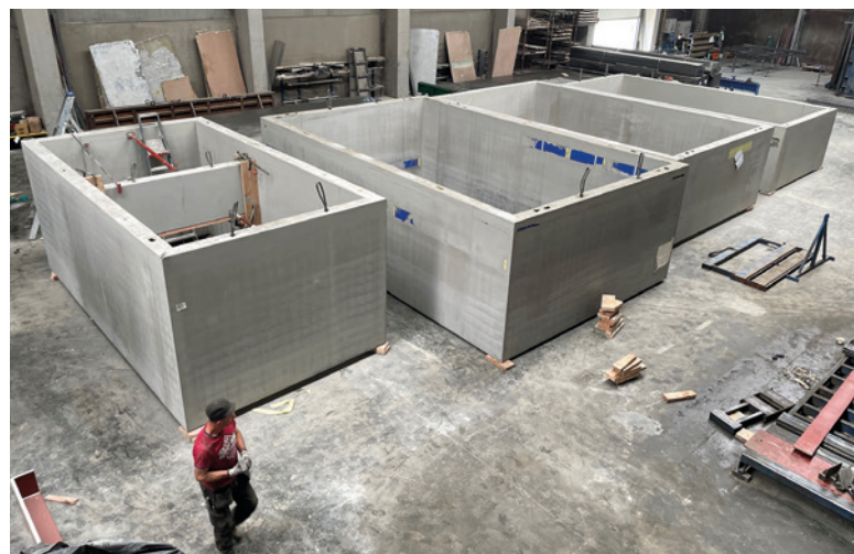
Stair cores right after demoulding, showing a fair-faced concrete finish
