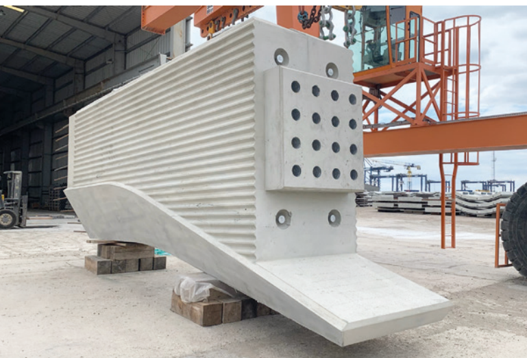
Precast piers 72 tons
