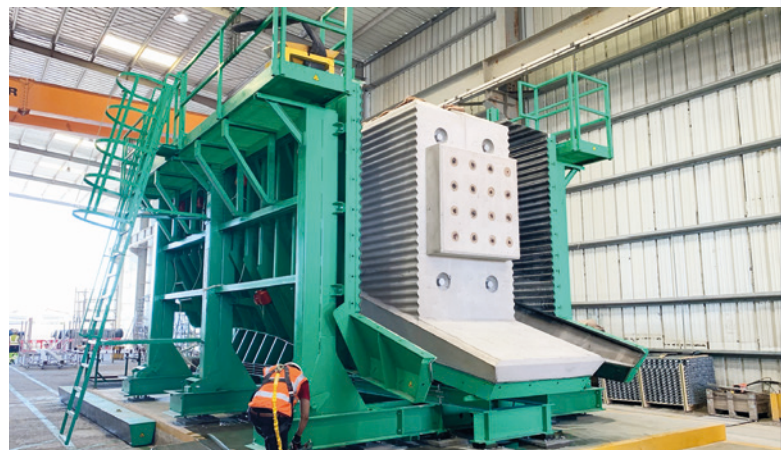
Production of bridge piers
