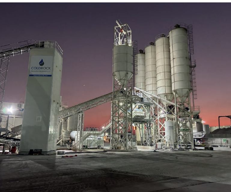
80-ton insulated aggregates cold weighing silo, ReadyMix Abu Dhabi, Mena Port UAE.
