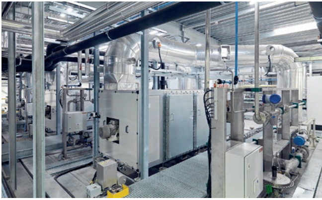
Chamber top with the process technology of the ProCarbonCure -system for CO 2 -negative facing bricks
