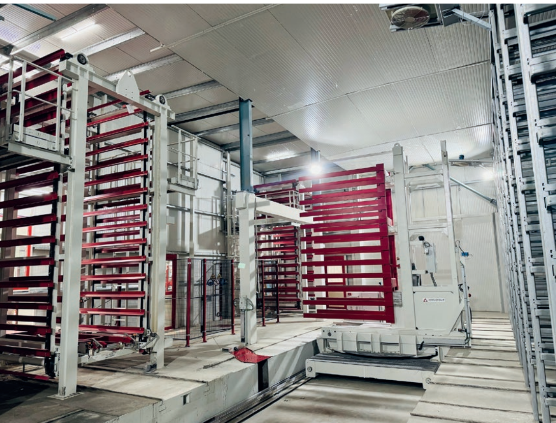
Curing with elevator and lowerator and finger car
