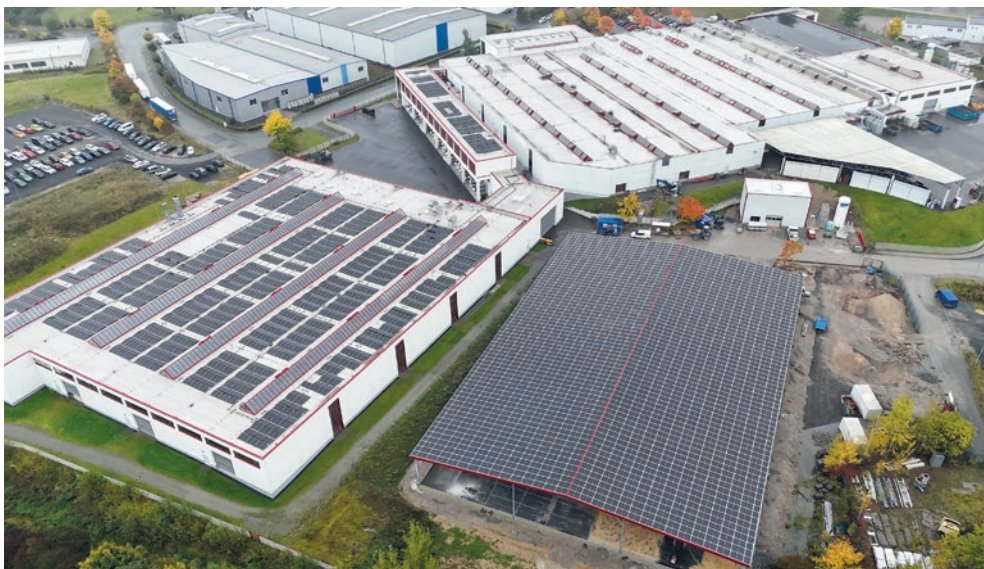
Kobra with 11 production halls and the new PV carport
