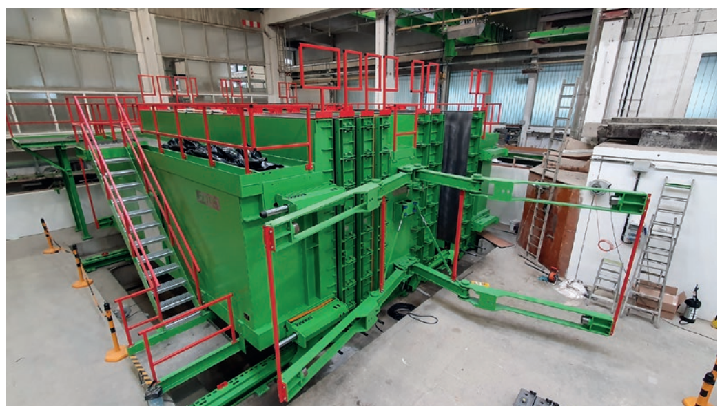
Battery formwork with tension arms for hydraulic clamping of pockets
